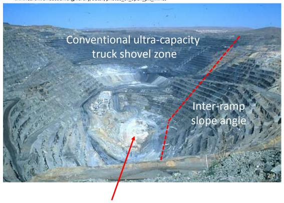
Potential zero-entry mining zone. Steep highwall, automated mining, less pushbacks necessary.
